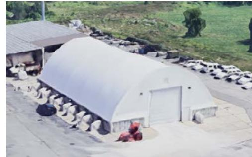
**Existing Condition:** The concrete blocks on the sides and rear of the shed have some gaps that need to be plugged, and a dry floodproofing system needs to be installed in front of the person and vehicle doors to protect against flooding incidents. There are several systems that could be implemented, as shown on this site:
